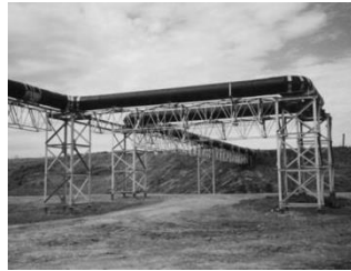
Figure 2.1: An expansion loop over the supports
