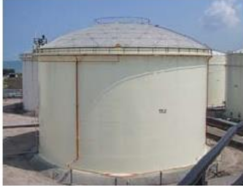
Geodesic Roof Tank (Dome-shaped Roof)
